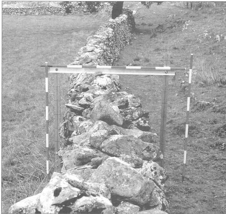
Documentary and field evidence indicates that this wall was standing in 1592. It was built in the mediaeval period as part of the infield boundary at Winstill, Upper Ribblesdale. It survives more or less as it was built apart from the loss of original topstones. The adjustable metal wall frame is an entirely new survey tool developed by Winstill Farm Visitor Centre to improve the recording of dry stone walls. Photo: Tom Lord.
